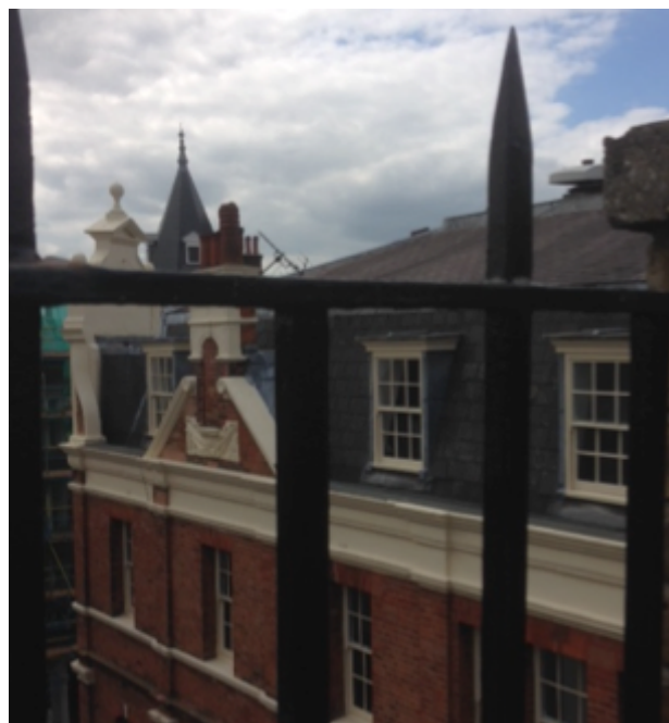
Fig. 7 Mansard roof extension to No. 28 Heath Street
