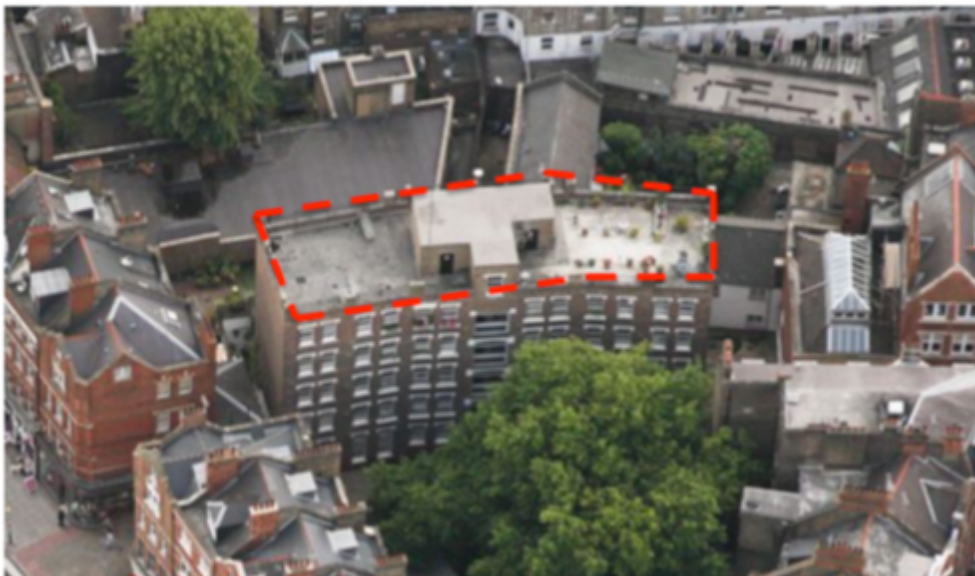
Fig. 2 'Birds-eye' view of site and surrounding context (looking south)
