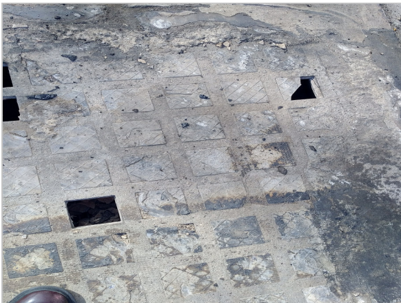
Fig 7. Pavement light condition following removal of asphalt.
