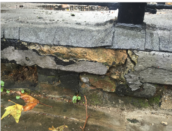
Fig 5. Image of beam bearing external.
