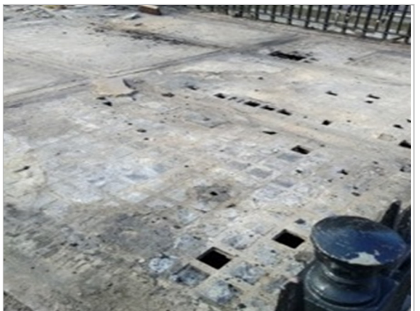
Fig 6. Pavement light condition following removal of asphalt
