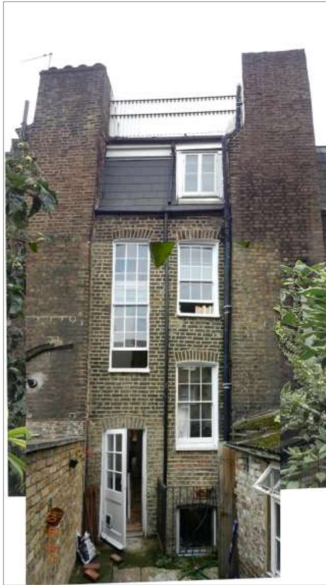
Figure 5: Composite photo of rear elevation
