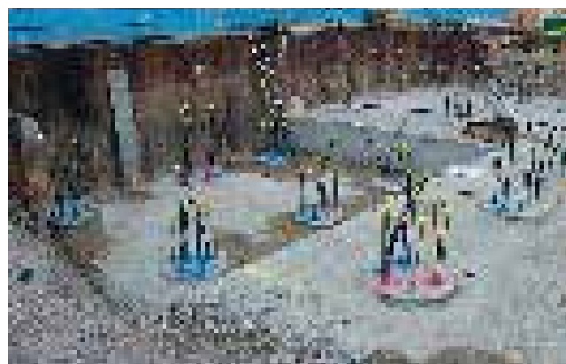
Energy piles within foundations of construction. Source: Geothermal International Italia
