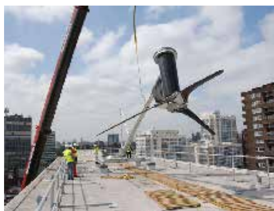
A building-mounted 6kW Proven wind turbine
