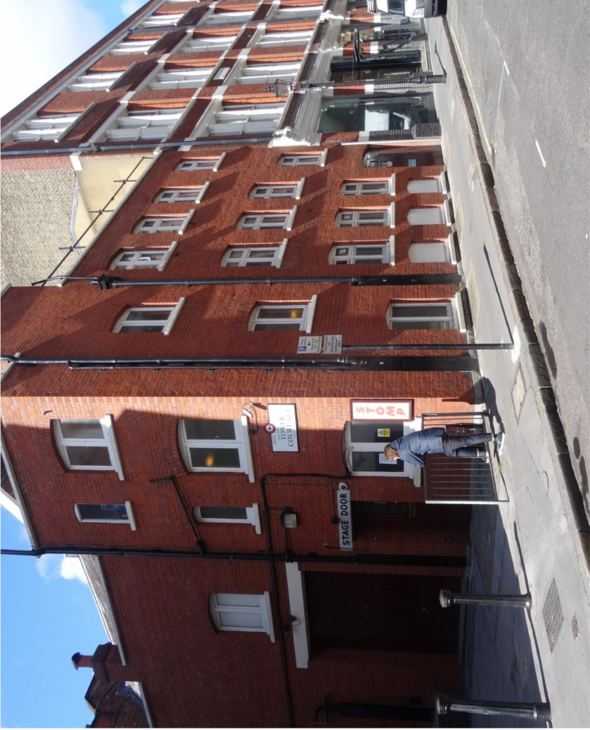
Rear elevation, dressing room windows, stair tower, stage door and get-in on left
