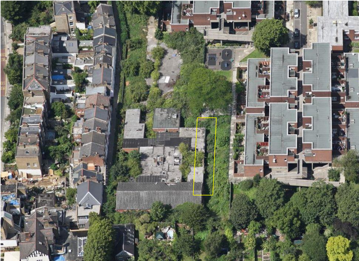
Aerial View showing approximate position of site Former BR Staff Club now demolished
