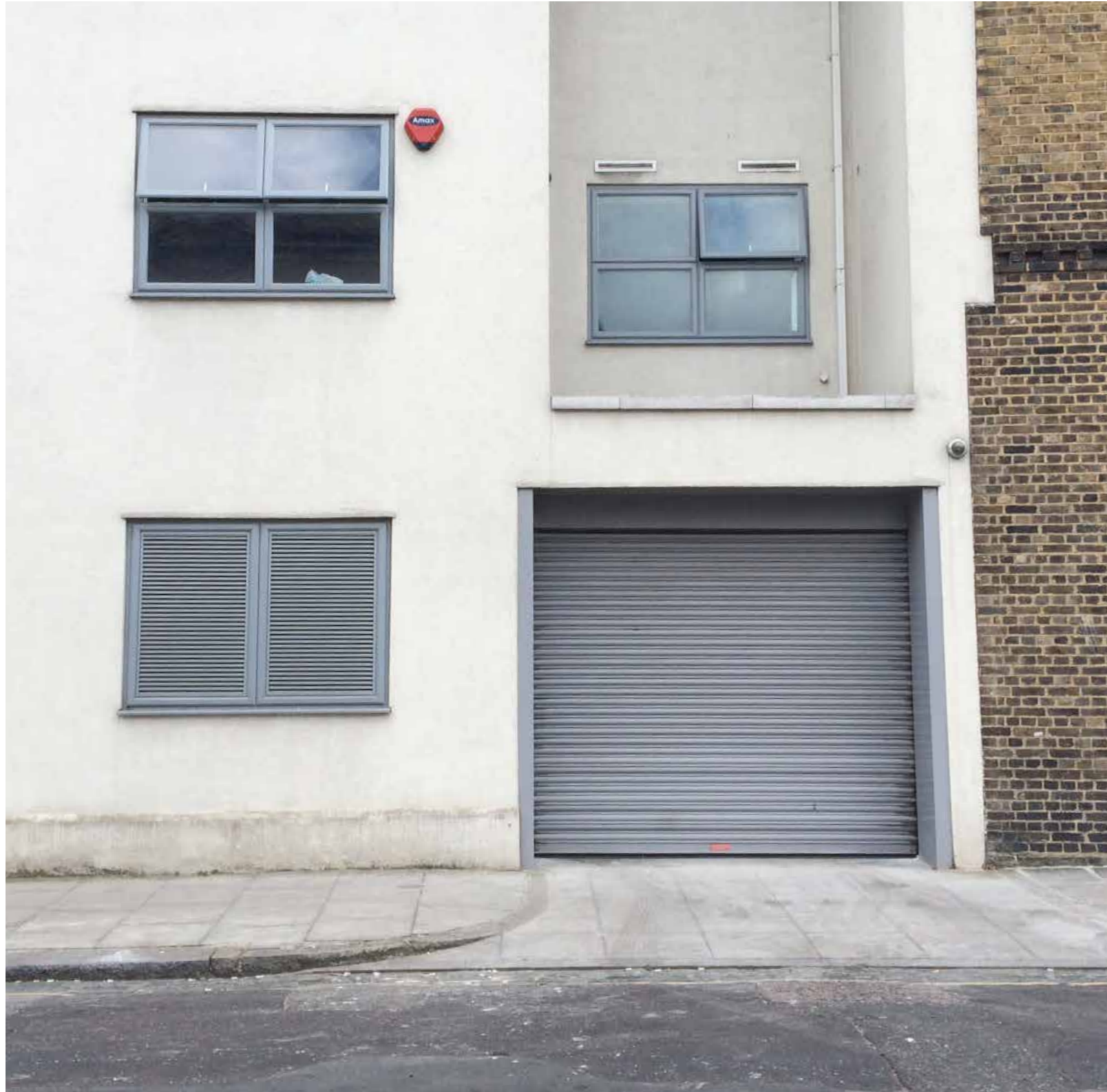
Existing garage shutter
