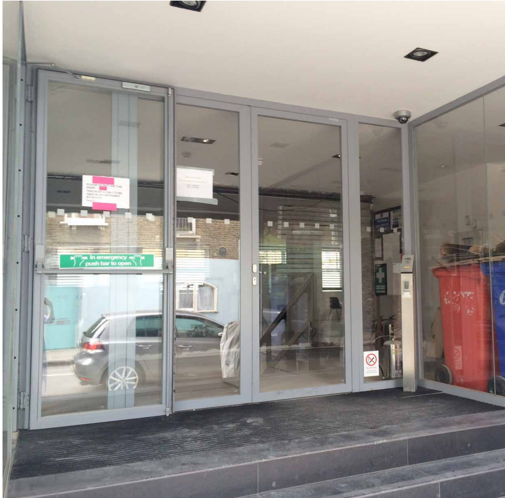
Existing entrance doors
