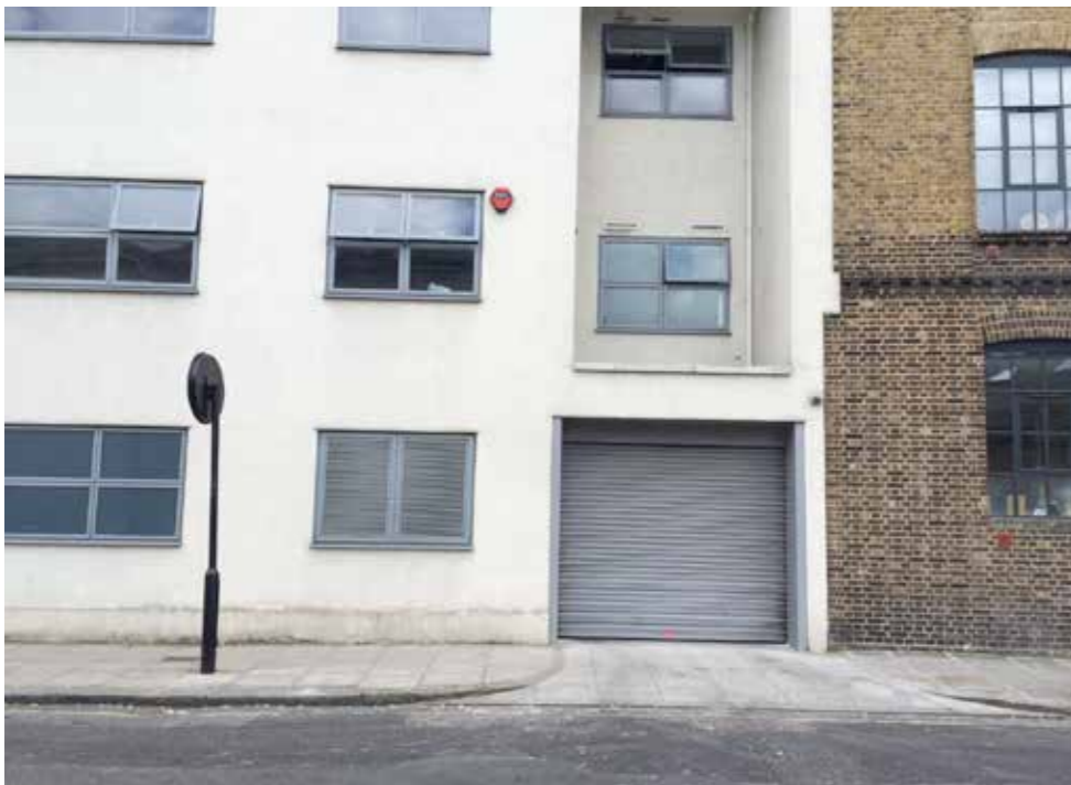
Wilken Street garage entrance
