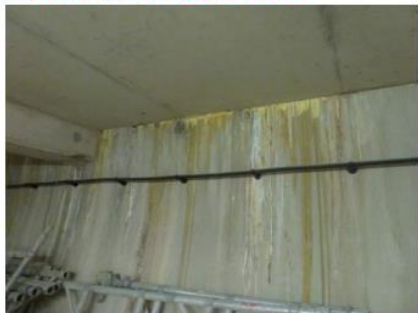
Figure 8.4.1: Water ingress recorded at junction between NLEB and Northern Line Lower Concourse Tunnel (West wall).
