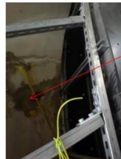
Figure 8.4.1: Water ingress recorded at junction between NLEB and Northern Line Lower Concourse Tunnel (West wall).
