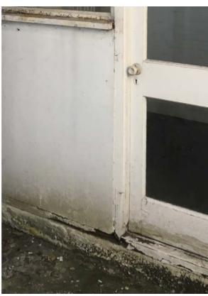
Non original glass/timber door with transom window and fixed side panel with top hung section
