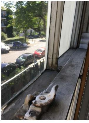
Original timber box frame and top sash, non-original bottom sash and beading
