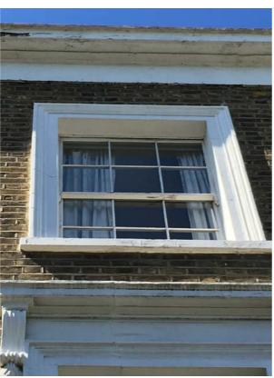
Flaking paint finishTop sash fixed shutSome rot to framing
