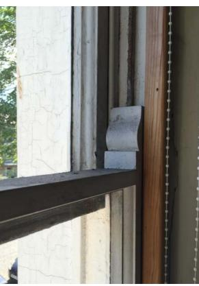
Original timber box sash frame and top Fair: sash, non-original bottom sash and beading
