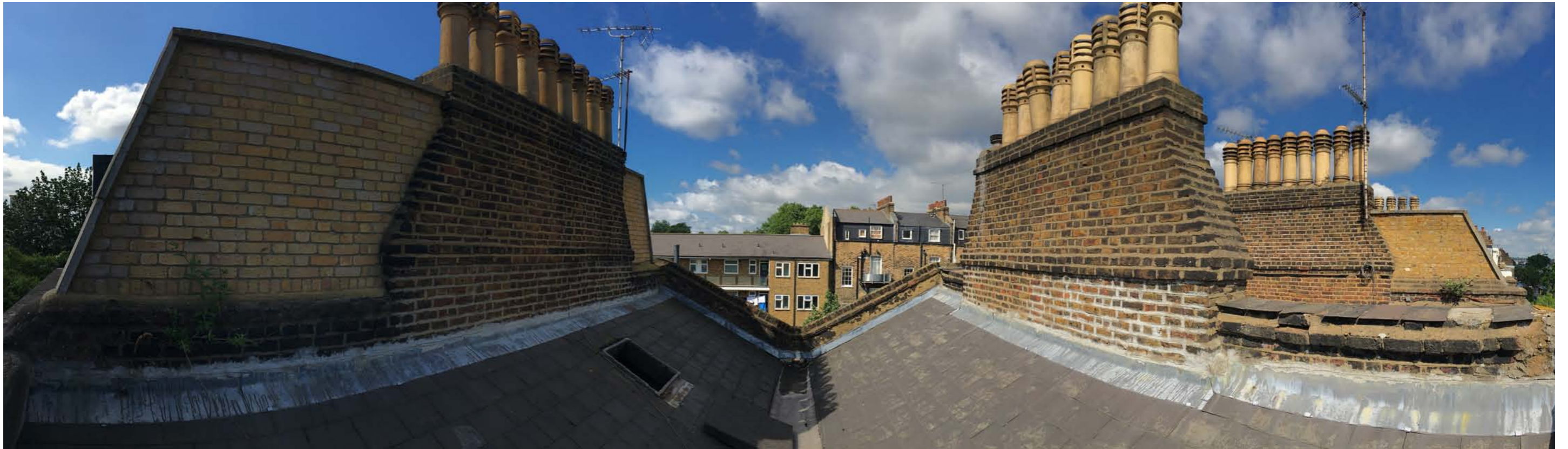
Panorama of the Existing Roof
