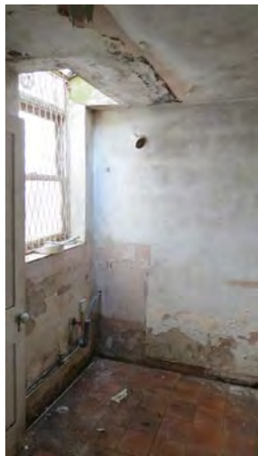
The coal-holes were knocked altered in the 1980's and now suffer from water ingress
