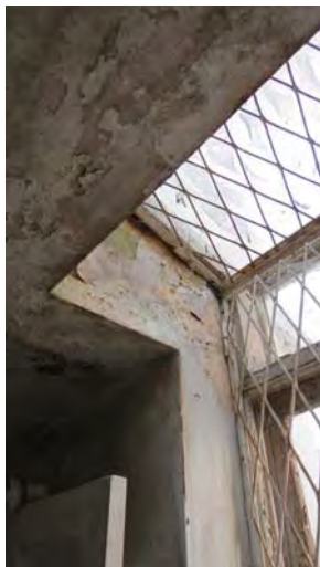
The coal-holes were knocked altered in the 1980's and now suffer from water ingress
