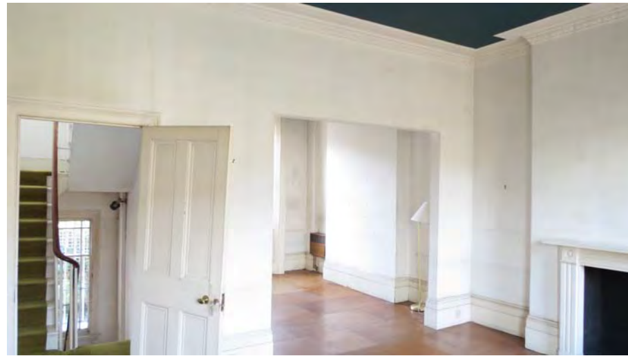
The spine wall on the first floor was opened up in the 1960's and is causing structural issues
