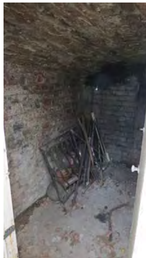
The coal-holes were knocked altered in the 1980's and now suffer from water ingress
