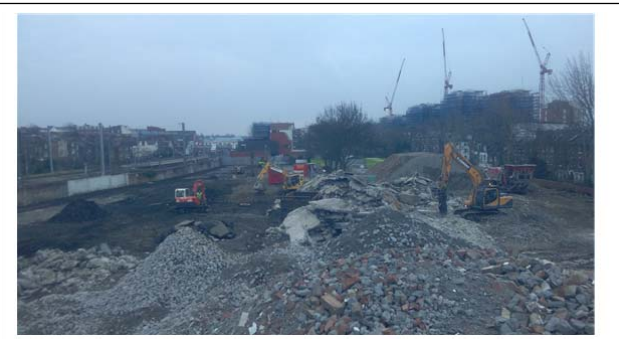
Picture 4: Activity of munching and crushing stone
