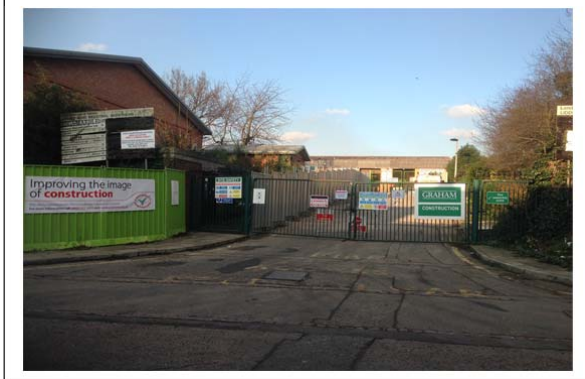
Picture 2: Site view of beginning of demolition
