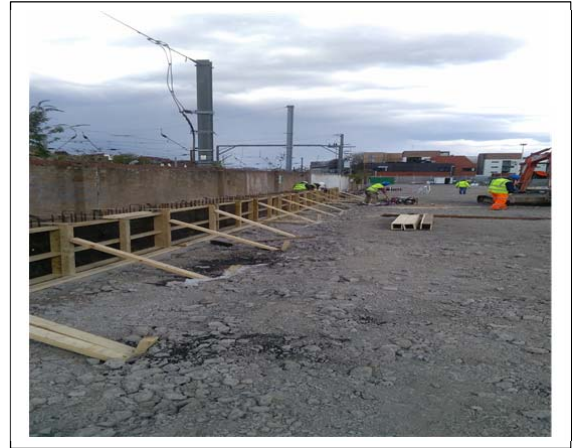
Picture 5: Shuttering for capping beam
