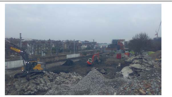
Picture 4: Activity of munching and crushing stone
