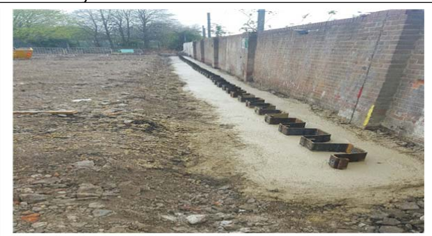
Picture 4: Sheet Piling to North West Boundary
