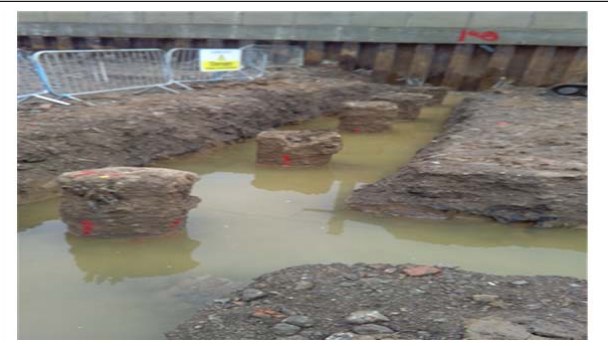
Picture 3: Slab development
