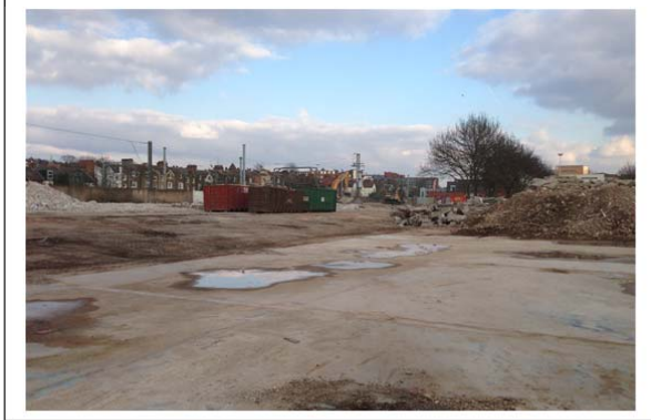
Picture 2: Removing slabs and foundation
