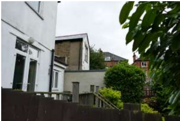
view of raised patio no. 3 and rear extension no. 1
