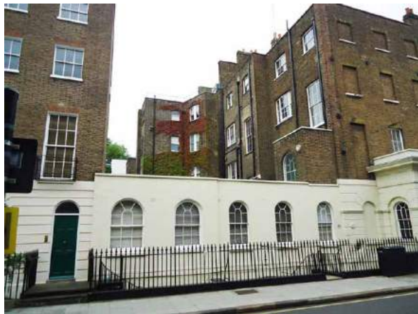
Fig. A2 View from Conway Street
