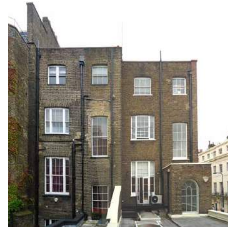
Fig. A4 View of rear elevation
