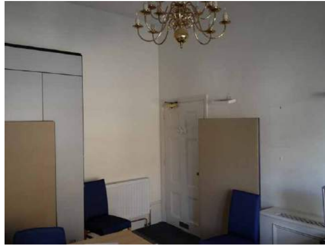
Fig. A34 1st floor - rear office
