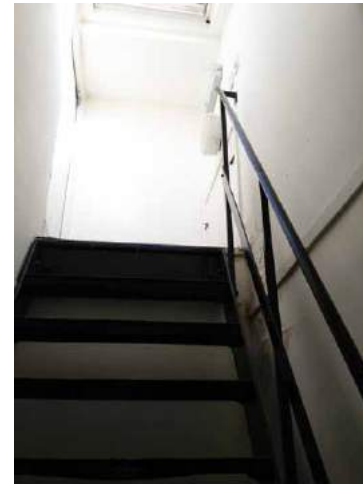
Fig. A44 3rd floor - stairs to roof
