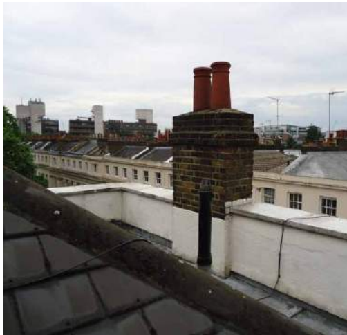
Fig. A50 Main roof
