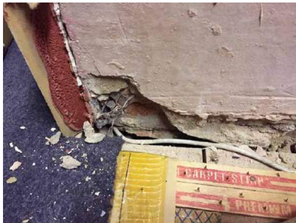
Fig. A27 Recent fletton brickwork and gypsum plaster to rear spine wall
