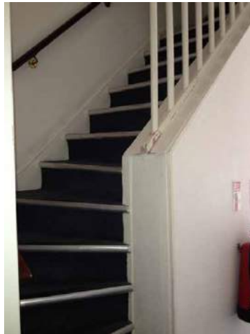
Fig. A39 2nd floor - stairs to 3rd floor
