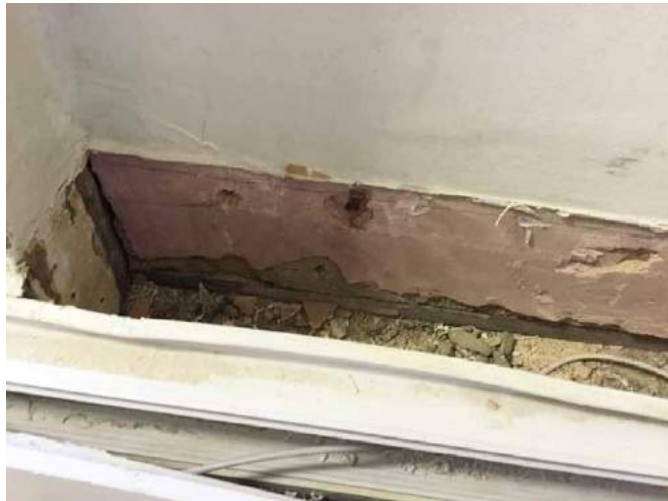
Fig. A24 Recent gypsum plaster to Conway Street facade
