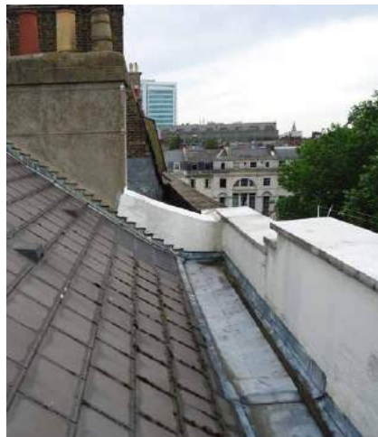
Fig. A51 Main roof
