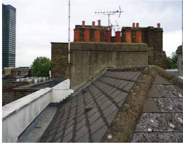
Fig. A48 Main roof
