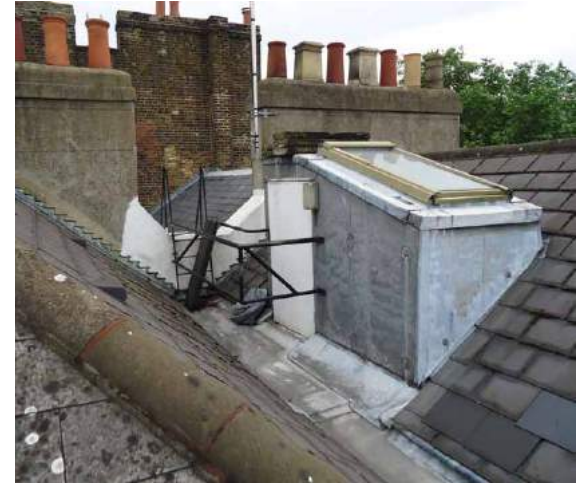
Fig. A49 Main roof
