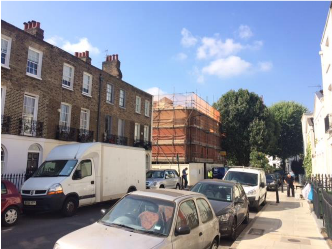
Photo 3: Current site photo - looking west at the site along Jeffrey's Street towards Camden Street
