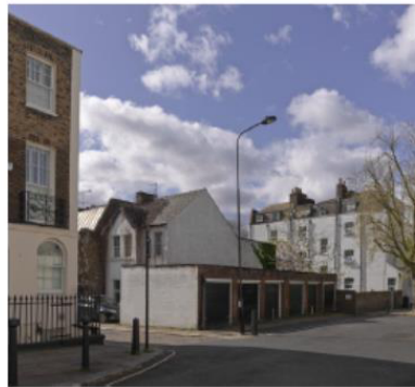
Southwest corner of garages Jeffrey’s Street/Prowse Place.
