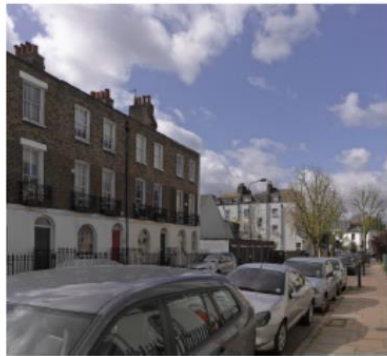
Site view looking southwest along Jeffrey’s Street
