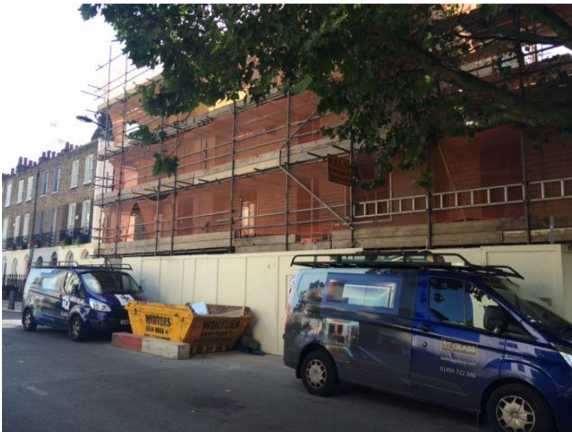
Photo 6: Current site photo – front elevation looking east along Jeffrey's Street.
