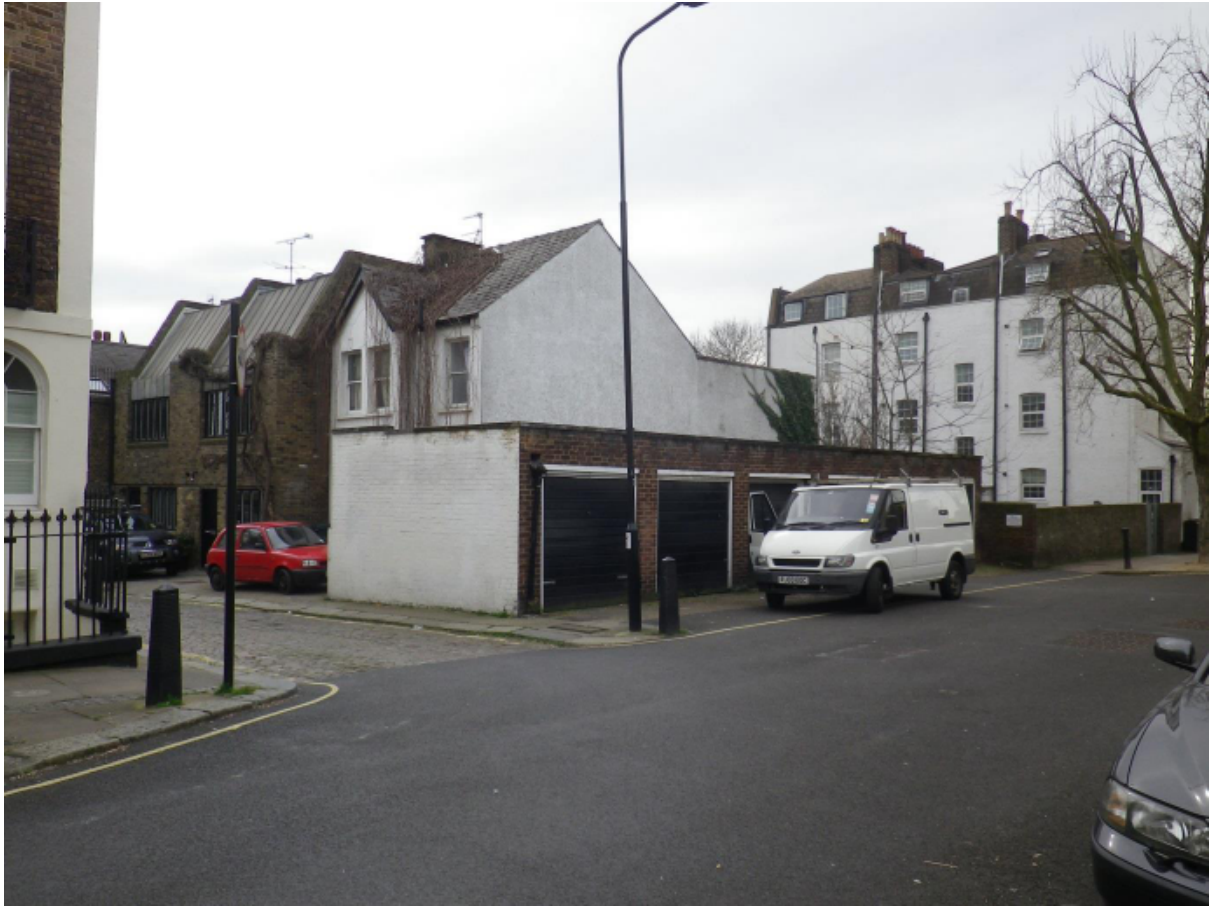
Photo 1: Photo showing the original garages on the site – pre development – looking west along Jeffrey’s Street.
