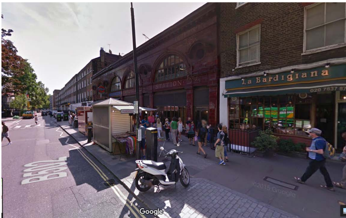
View of Bernard Street and site from Russell Square and Woburn Place
