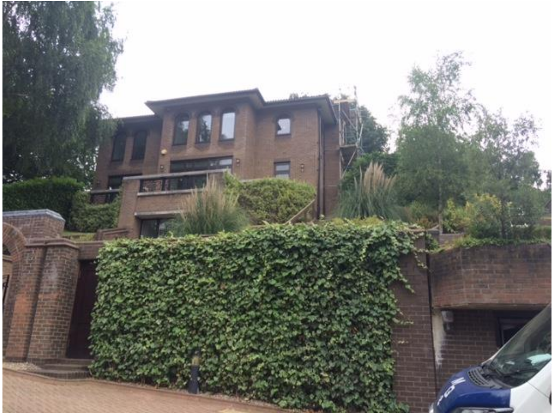
Photo 1 - Front elevation view from Highfields Grove
