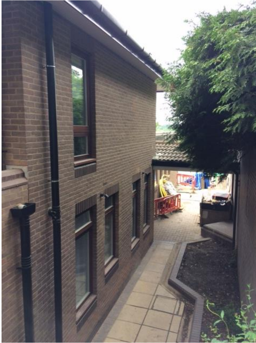
Photo 6 - Side elevation of neighbour at no. 5 - showing side windows and existing high hedge with the application site.
