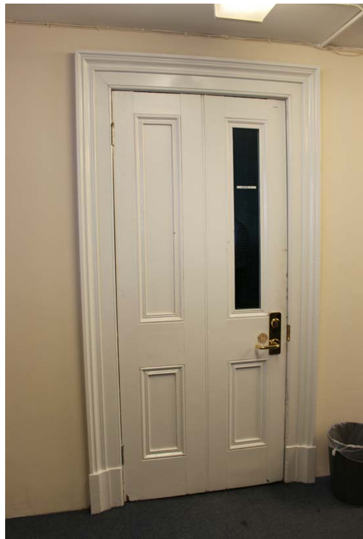
EXISTING DOOR TO NORTH SIDE OFFICE TO BE REPLACED WITH FIRE RATED DOOR
