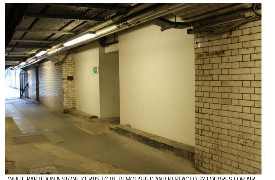
WHITE PARTITION & STONE KERBS TO BE DEMOLISHED AND REPLACED BY LOUVRES FOR AIR
