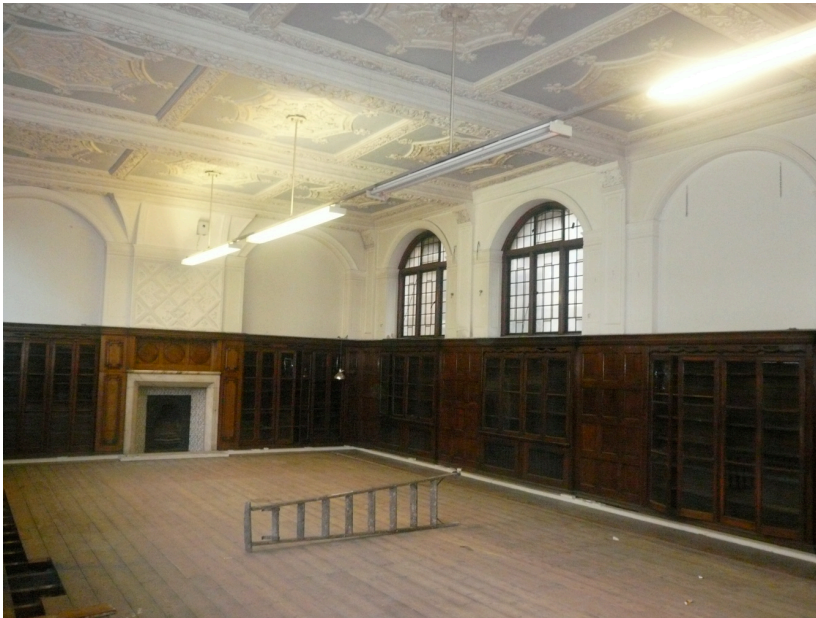
Figure 2 Room 2.07 as existing, showing fireplace, display cabinets, arched windows and decorated coffer-effect ceiling.
