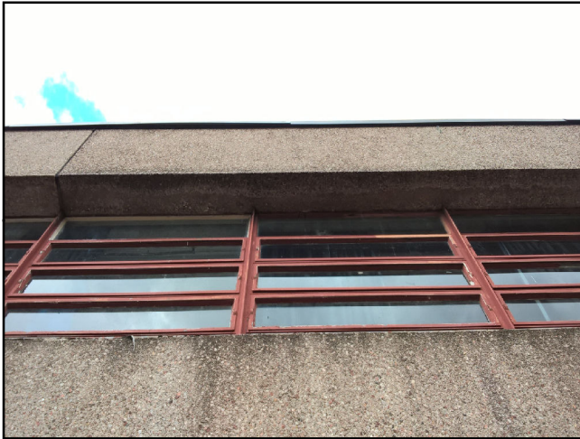
Photograph 1: Lifted fascia board in courtyard of building B5.
