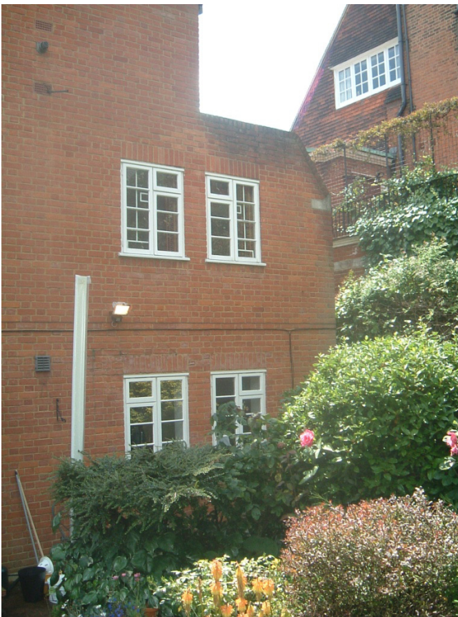
2. View of the dining room to the right
