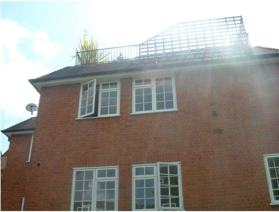
3. View of the rear at high level
