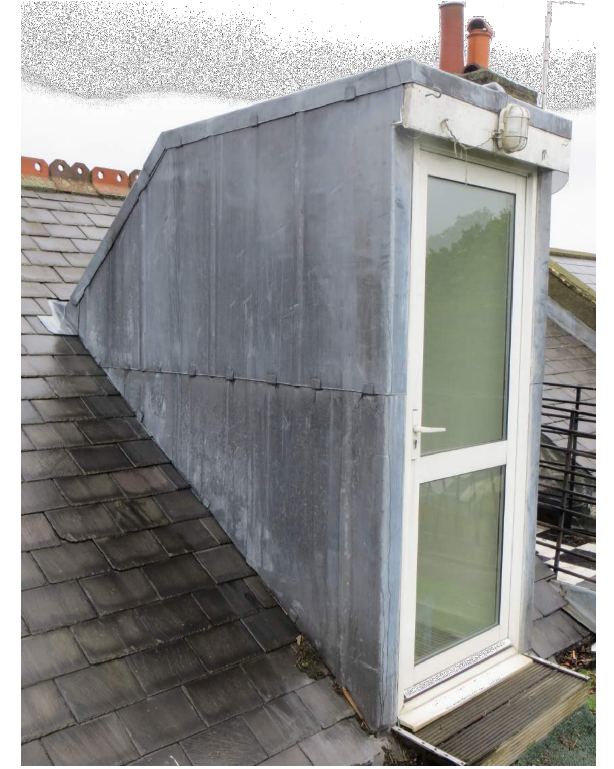
4. Rear Door to Roof Terrace
