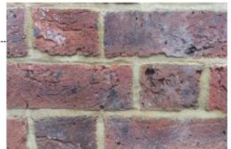
Sample of brickwork washed, repaired and repointed
