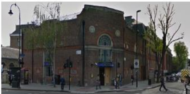
Brickwork and masonry work to existing facades to be cleaned and repair where necessary. Design to be in accordance with consented elevations.
