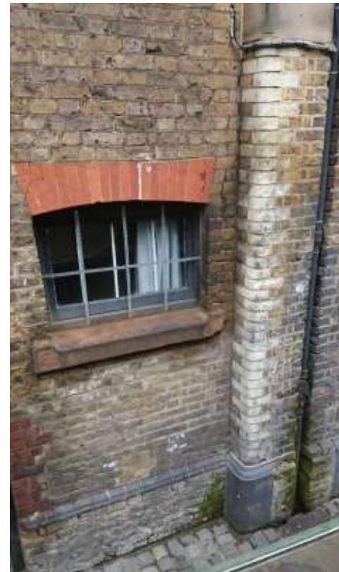
Figure 11: Unit 87 (South elevation) – metal straps fixed across window
