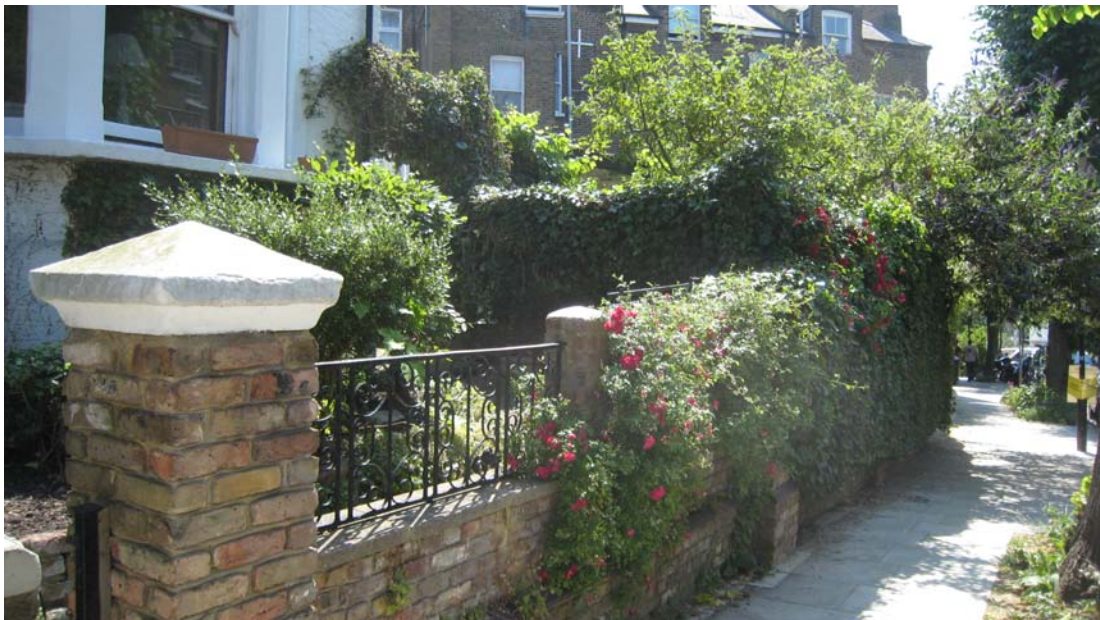
Image 2: Front Wall to 1 South Hill Park
