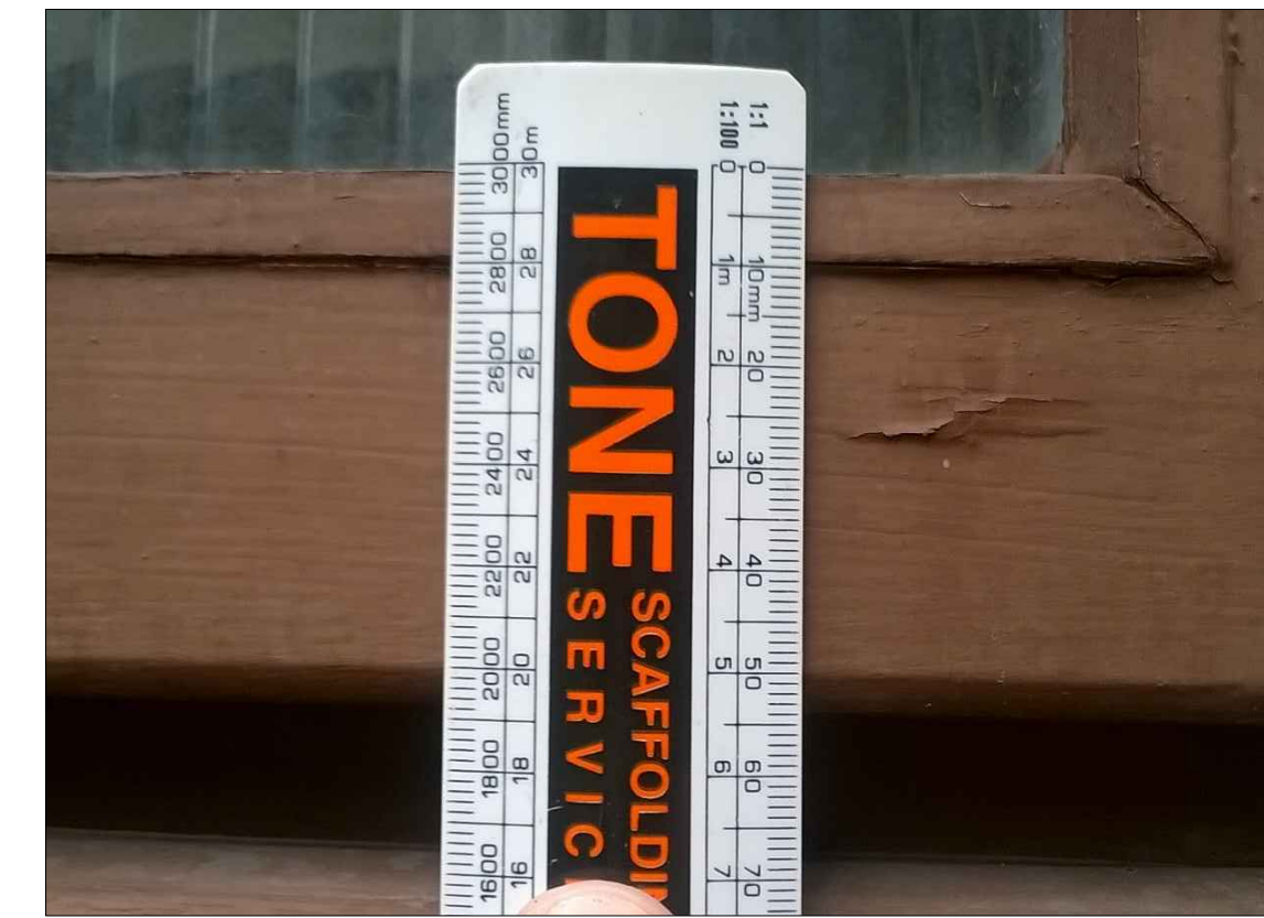
Existing window frame - thickness 55mm.
