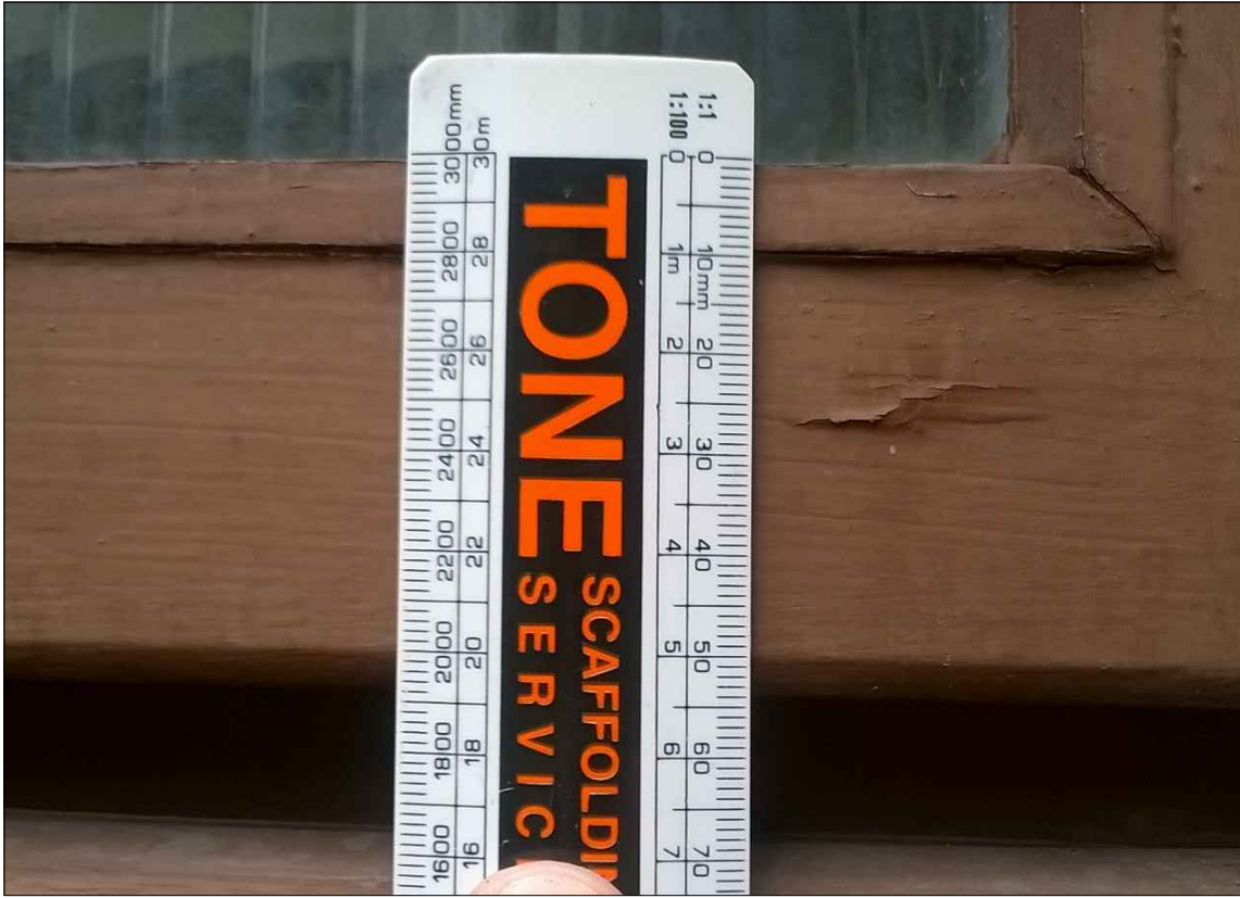
Existing window frame - thickness 55mm.
