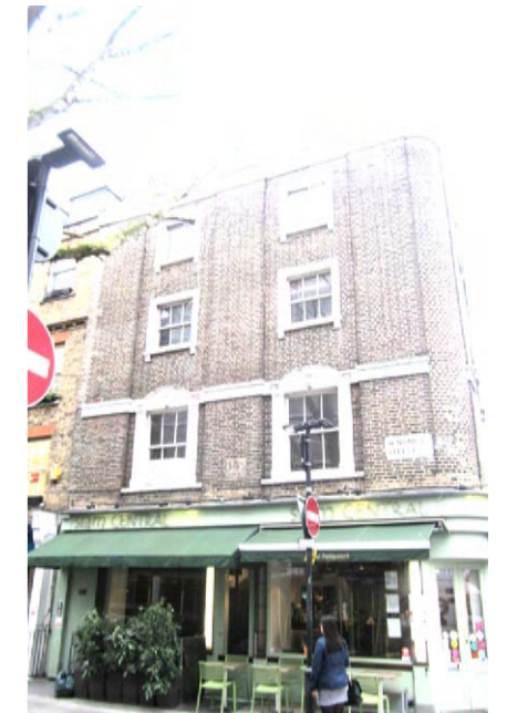
Figure 4: View from Windmill St.
