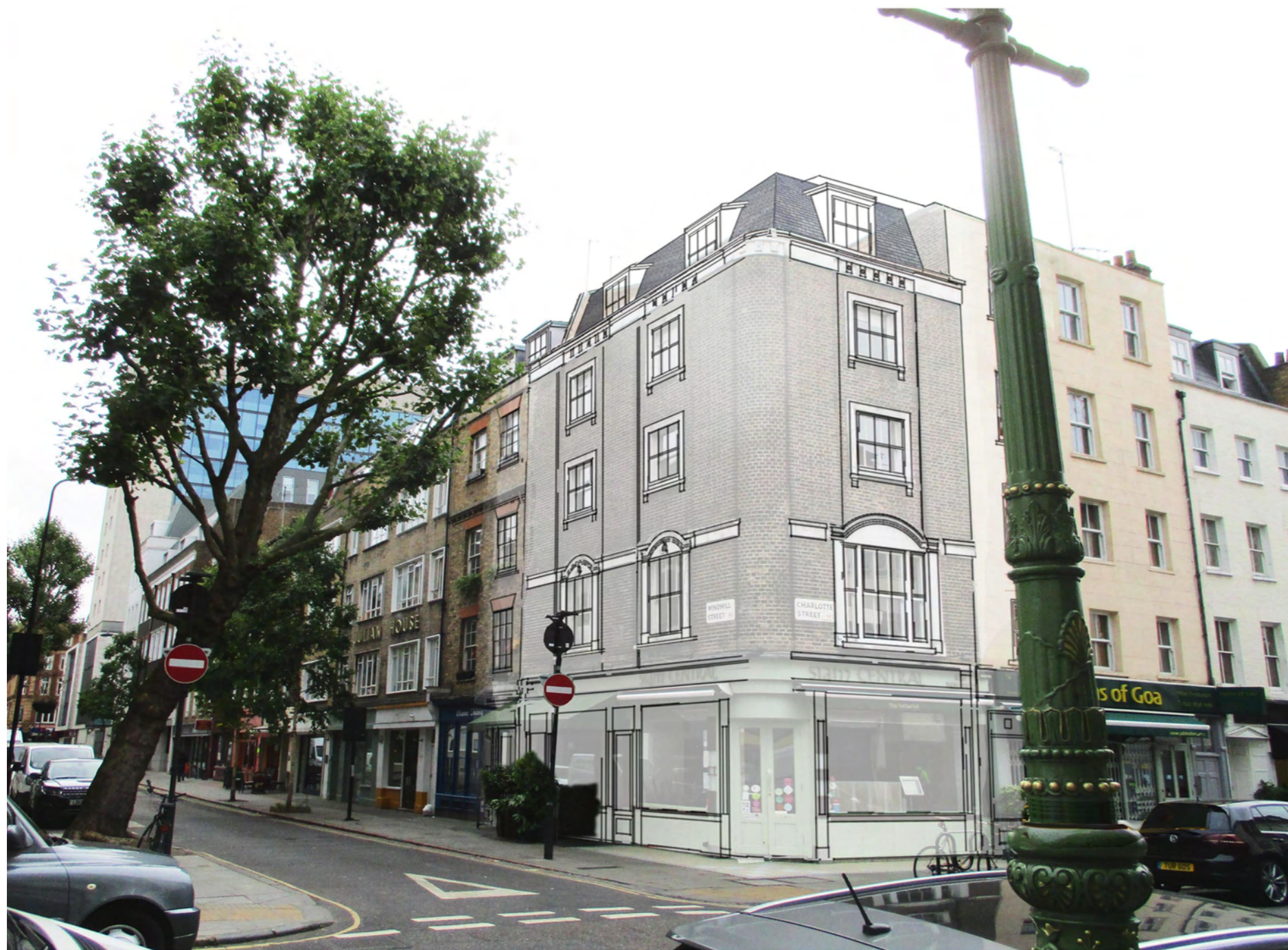
View looking east from Charlotte St.
