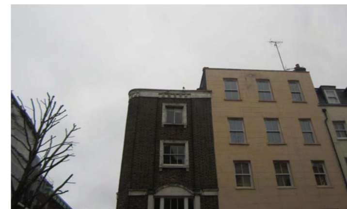
Figure 5: Neighbouring no.12 Charlotte St rising an additional storey.
