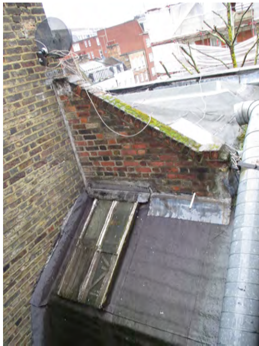
A EXISTING PHOTOGRAPH A
