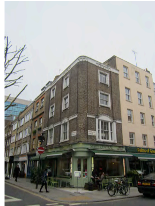
F EXISTING PHOTOGRAPH F
