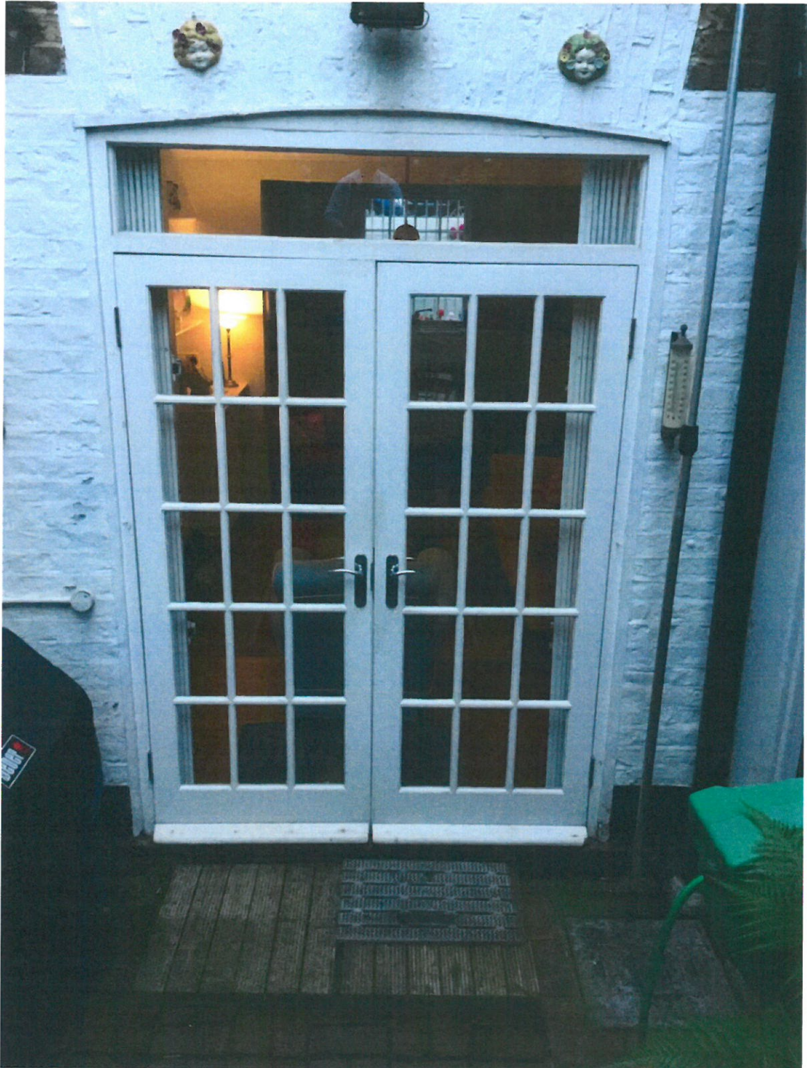
11 ROTHWELL STREET – EXISTING FRENCH DOORS - EXTERNAL
