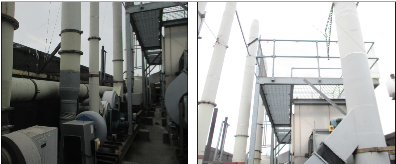
Photo 2 and 3: The UCL Roberts Building Roof (showing services and raised platform).
