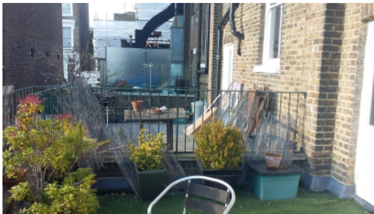
Existing roof terrace (looking west)
