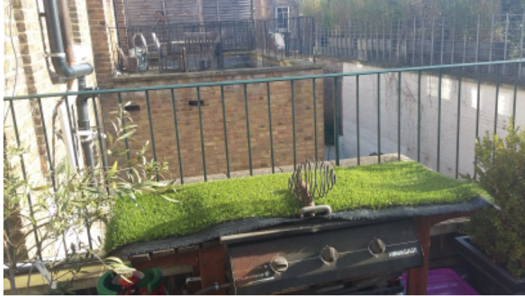
Existing roof terrace (looking east)
