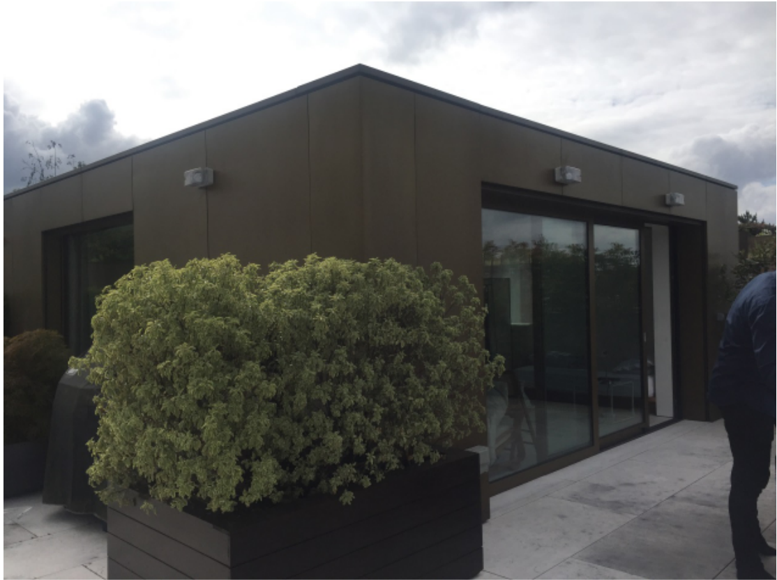
Photograph 5- View of the existing sunroom.
