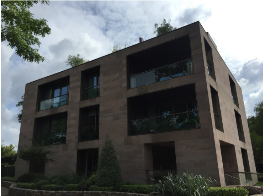
Photograph 1 – View of front elevation of Block A from application site.
