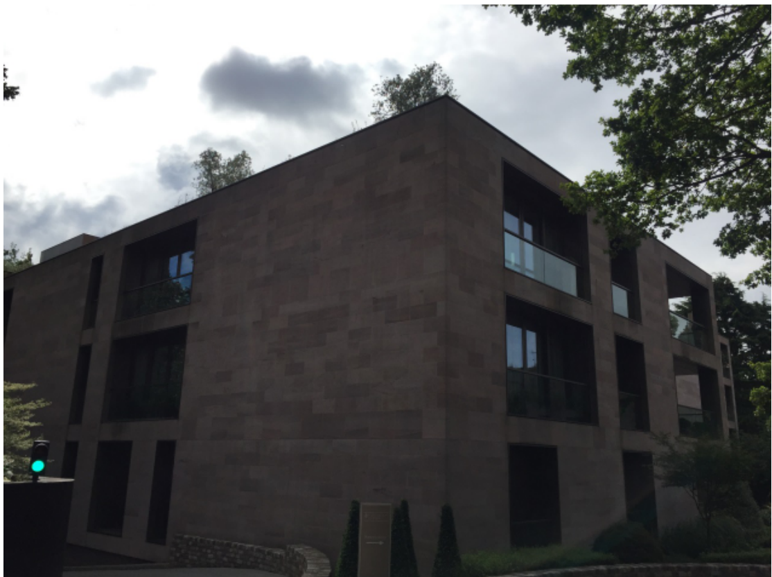
Photograph 2 – View of front and side elevation of Block A from application site.
