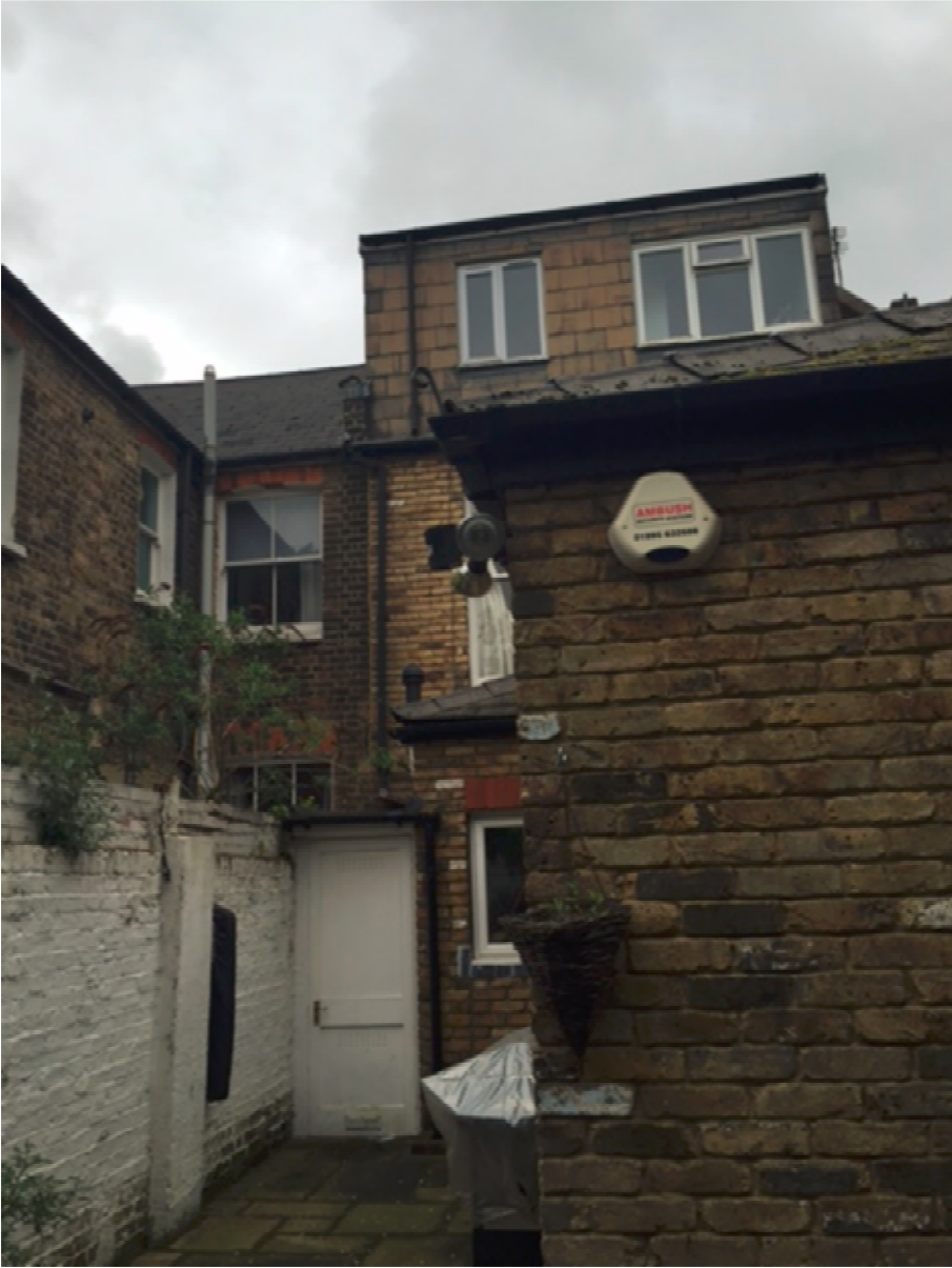
Photo 1 – Location of infill extension
