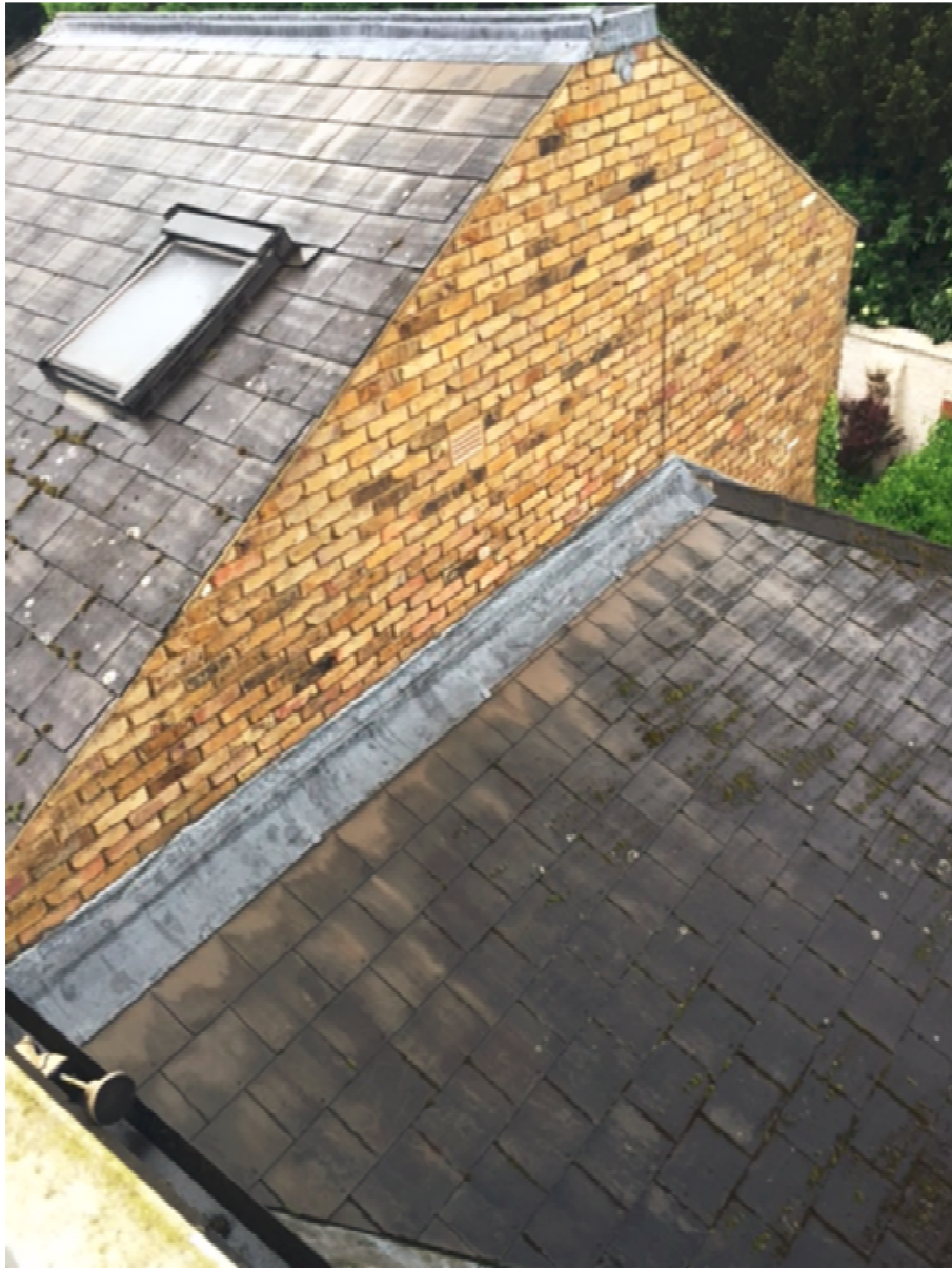
Photo 3 – View from first floor rear window to location of extension
