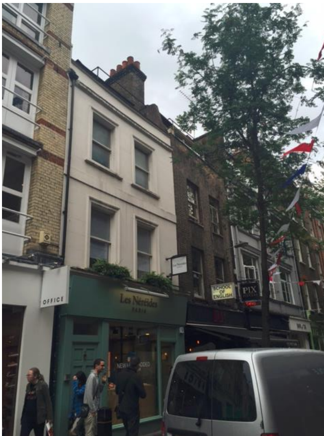
Photo 2 – Close view of Gr II Listed Building (no.61 Neal Street) and no.63 Neal Street
