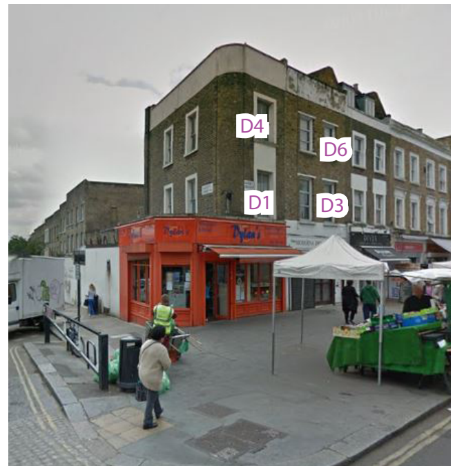
Assessed windows at 72 Queens Crescent
