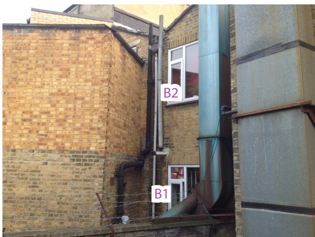
Assessed windows at 143 Queens Crescent
