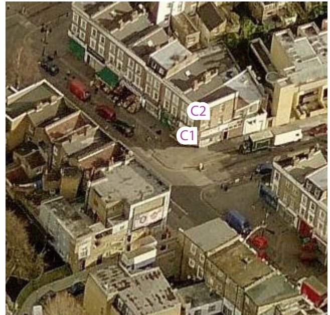
Assessed windows at 74 Queens Crescent
