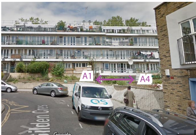
Assessed worst-case windows at Community Centre
