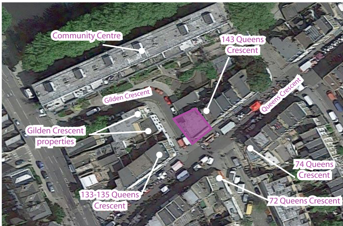
Aerial view of surrounding areas of the proposed development at 139-141 Queens Crescent (approximate site area highlighted in pink).
