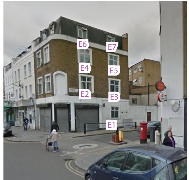
Assessed windows at 133-135 Queens Crescent
