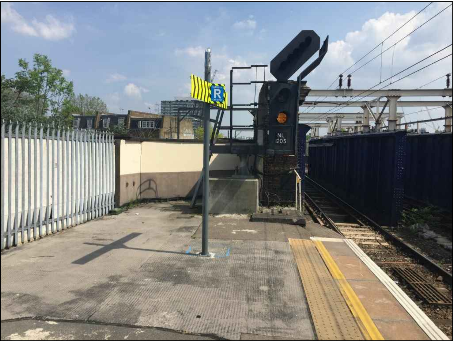
PLATFORM 2 (STRATFORD END) FENCE HEIGHT 1250mm DUE TO SIGNAL SIGHTING
