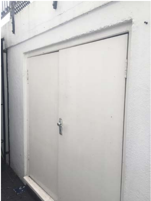
Water Tank Store
