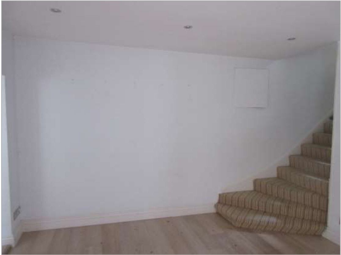
4e: Internal basement view towards stair
