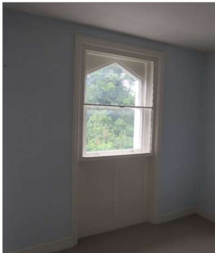
4s: Window, second floor front bedroom
