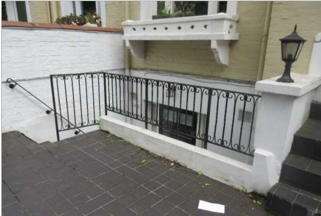
4a: Front garden, showing modern tiling, light fittings and railings to basement area
