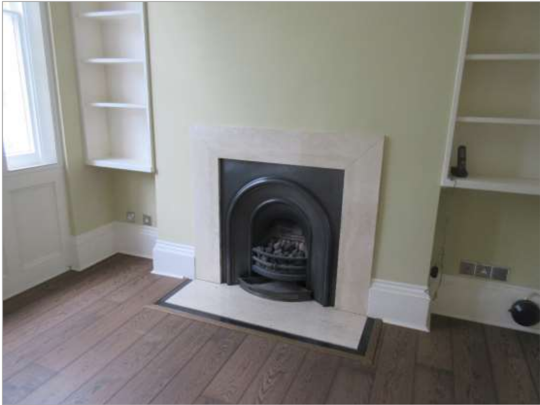
4n: Ground floor front room, salvaged C19 fireplace insert with modern surround
