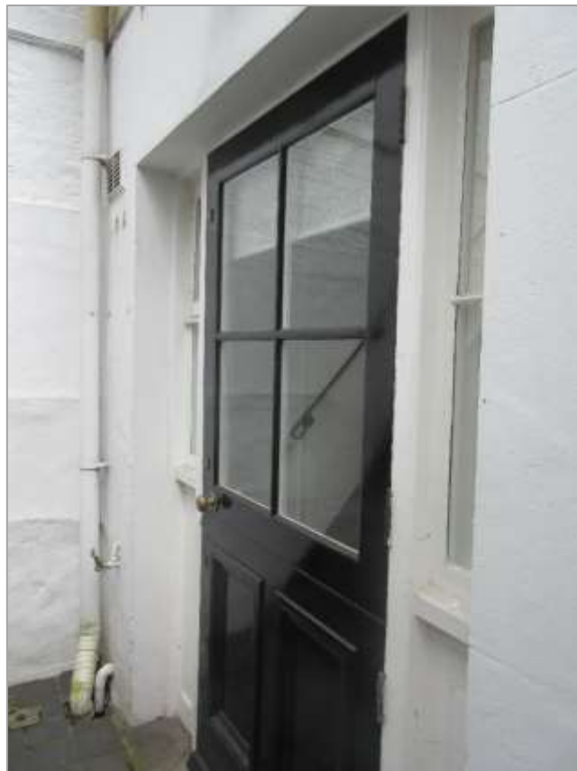
4b: Door to basement area
