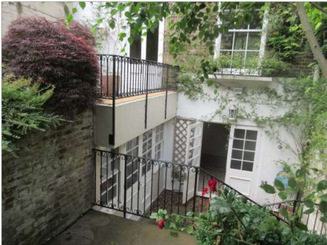
4d: Rear basement area
