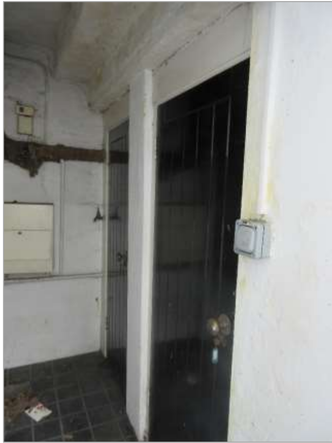
4c: Doors to basement vaults
