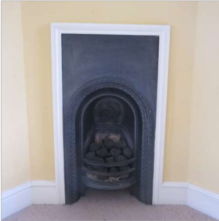
4r: Corner fireplace, second floor rear bedroom
