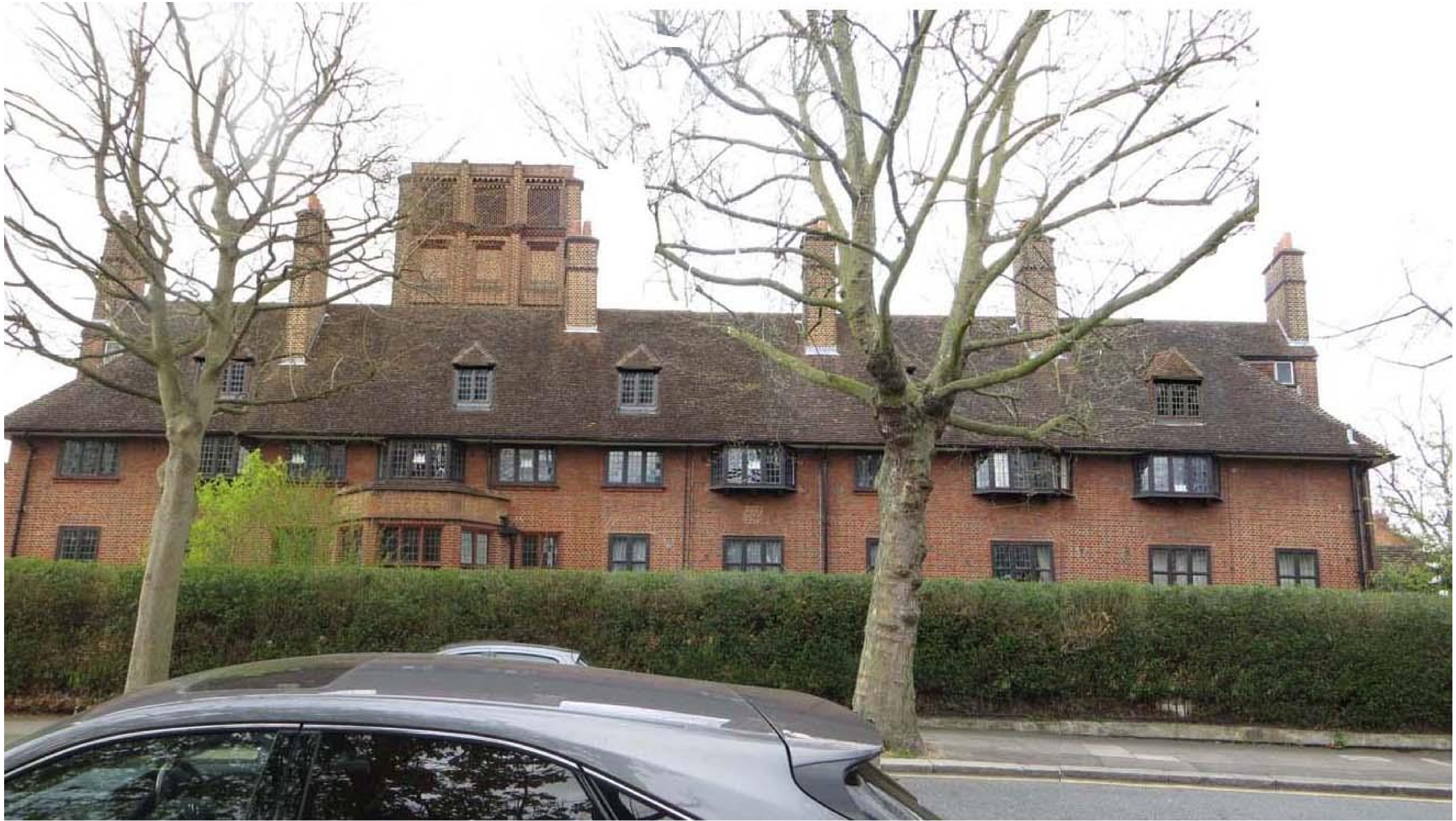
IMAGE SHOWING 5 DORMERS ON THE SOUTH ELEVATION.
