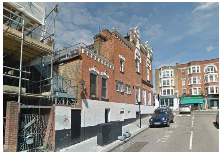
Rear View, Ravenshaw Street.
