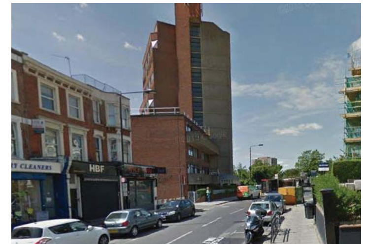
West View, 40-42 Mill Lane.
