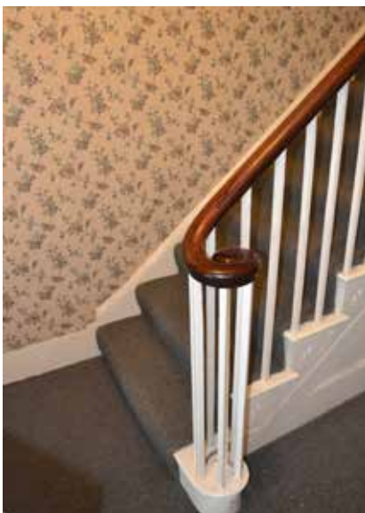
20. Staircase at Ground Floor. DIA
