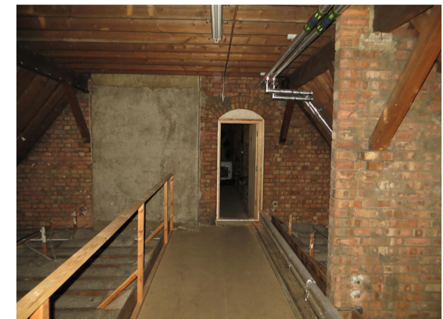
SOUTH ATTIC SPACES PUT SUSTAINABLY TO RESIDENTIAL USE
