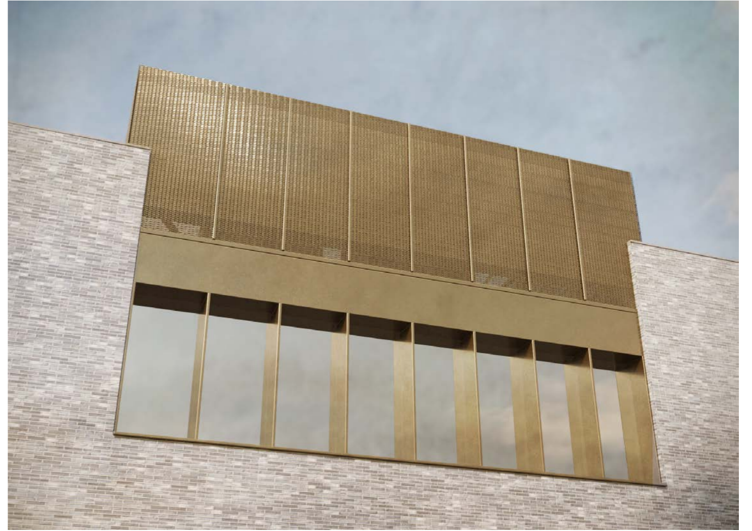
indicative view of plant screen on south elevation PPC Expanded aluminium mesh - RAL 7008 - 30% gloss
