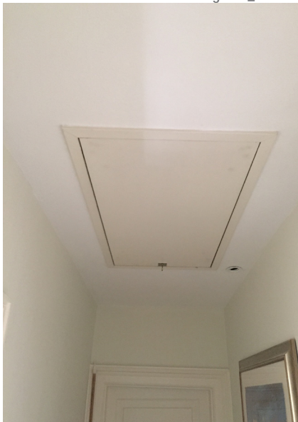
Fig. 12_ Corridor with ceiling hatch
