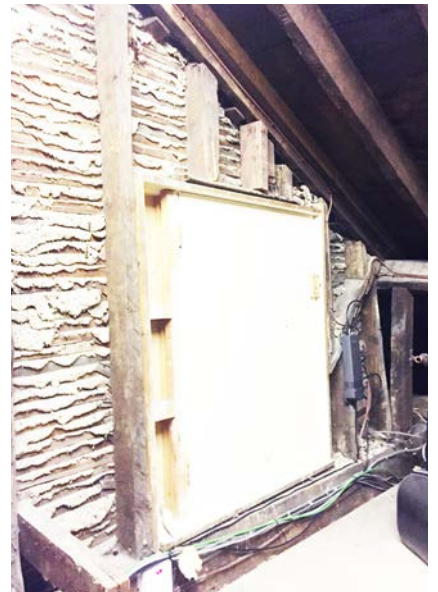
Fig. 14_ Loft hatch to balcony
