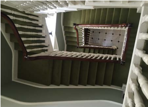
Fig. 11_ View down stair well
