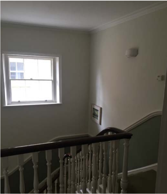
Fig. 10_ Stair well at top floor
