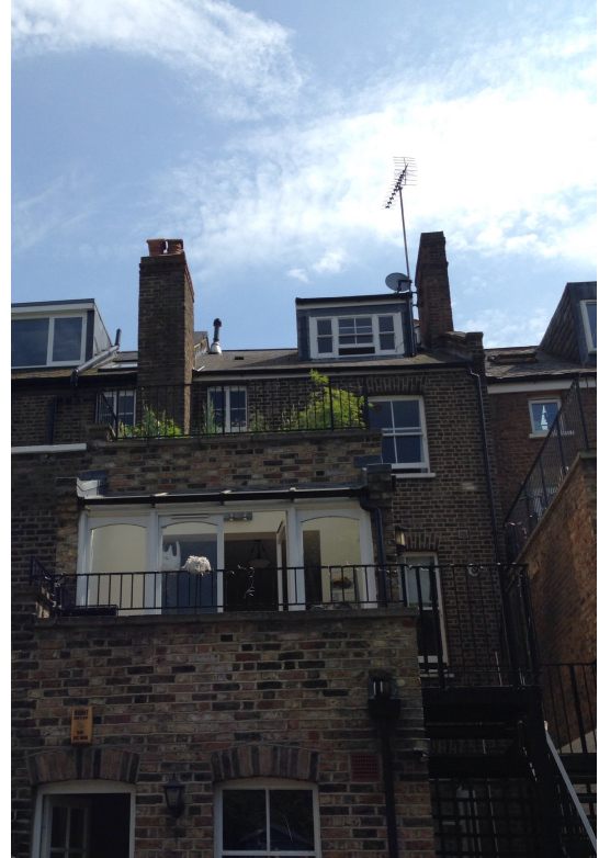
Photo of existing rear elevation and dormer
