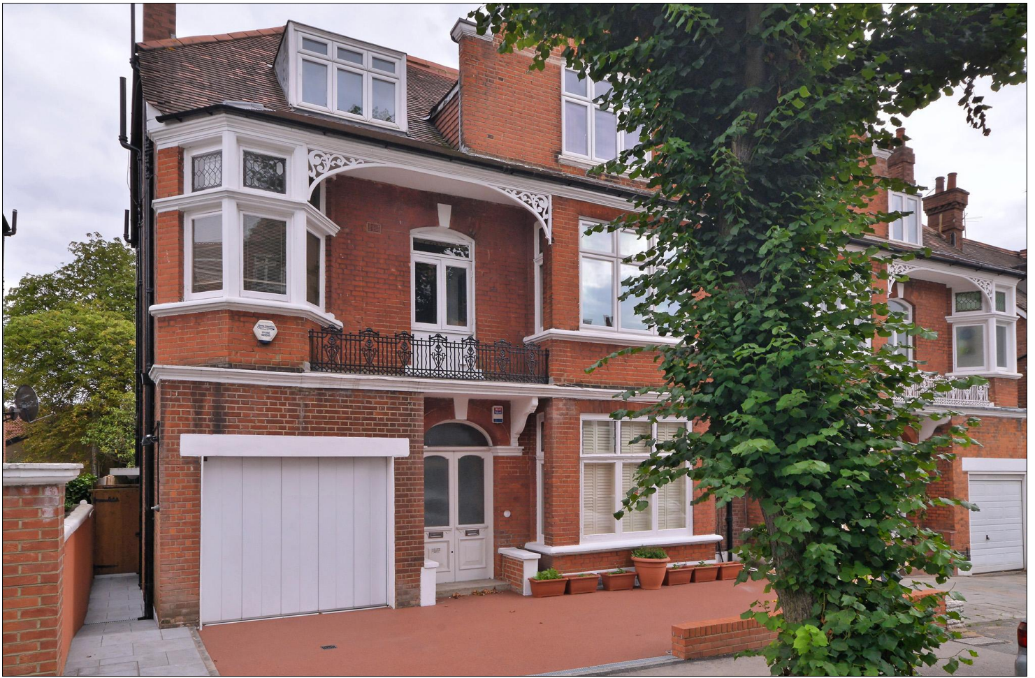
Figure 1: External photo of 16 Crediton Hill showing garage door.
