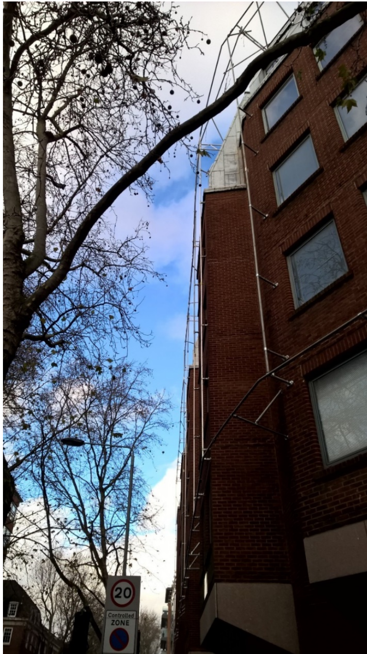
Figure 2: Tree 2 and its relationship to the building. Tree 1 is in the background where the degree of separation from the building can be seen
